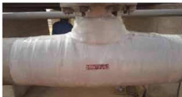
Wrapping completed (12 layers) & ID plate installed ●
