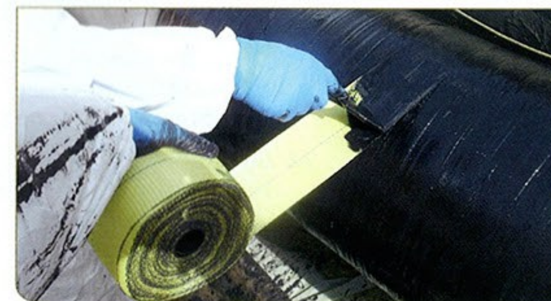
Application of REINFORCEKIT 4D on the pipe
