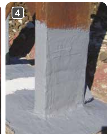
4 Protective coating application
