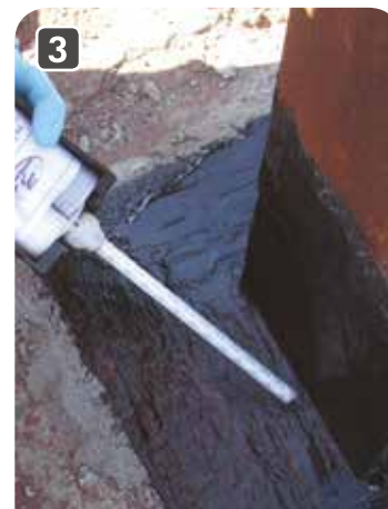
3 Waterproofing by elastomeric resin application
