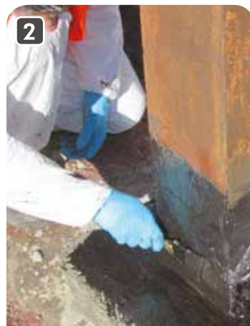
2 Epoxy resin application for beam/concrete protection
