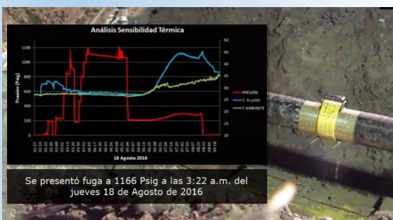
Figure 4: Pressure test for 10mm hole → leaks at 1166 psi
