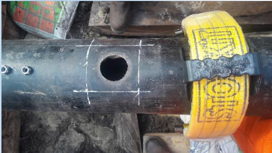
Figure 1: Straight line with the defect
