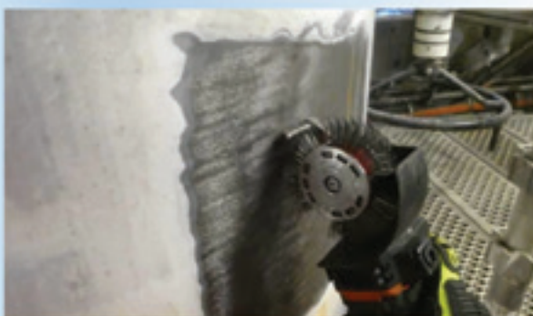
Fig. 3: Surface preparation using Bristle Blaster®
