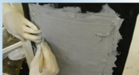
Fig. 4: Composite patching on progress
