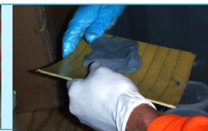
Primer & composite plate with filler application (steps 1 & 2)
