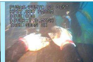
Tape impregnation using BOBIPREG & R4D-S wrapping (step 4)
