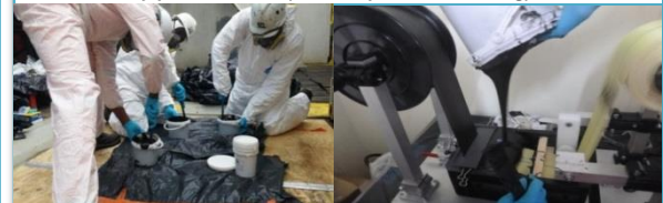
Mixing of the resin and tape impregnation using BOBIPREG (3X specific tool) to avoid lack of resin.
