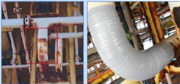
Fig. 3-4: Elbow reinforcement (before/after)
