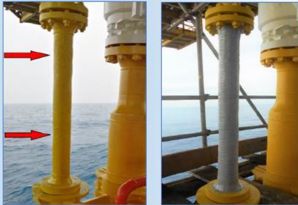
Fig. 1-2: Straight line reinforcement (before/after)
