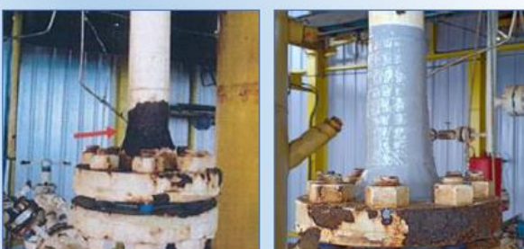
Fig. 7-8: Flange reinforcement (before/after)
