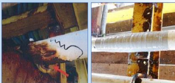
Fig. 5-6: Pipe on support reinforcement (before/after)
