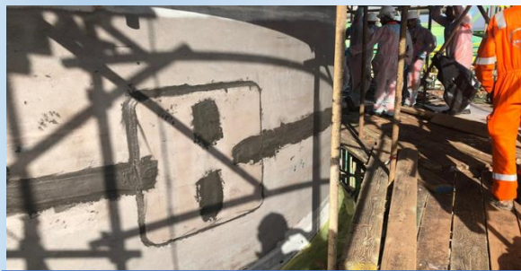
Fig. 2: F3XS1 application on weld
