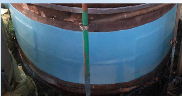
Fig. 6: Wrapping completed (4 layers)
