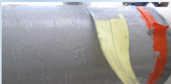
Fig. 3: Wrapping in progress
