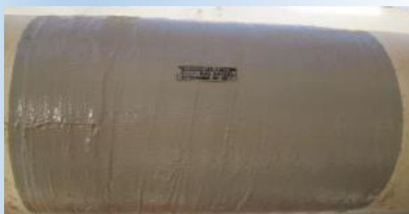
Fig. 4: Wrapping completed & Identity plate installed
