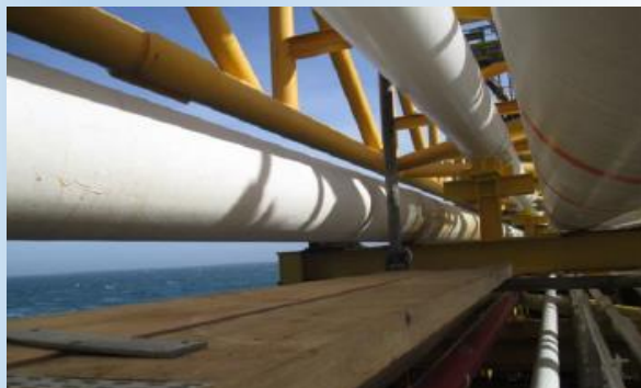
Fig. 1: Working conditions – View of scaffoldings
