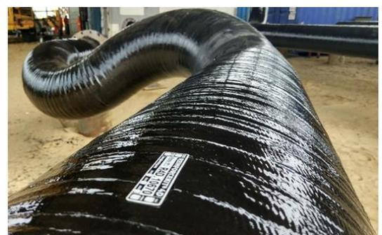
Figure 5: Reinforced protection finalized with reference plate installation
