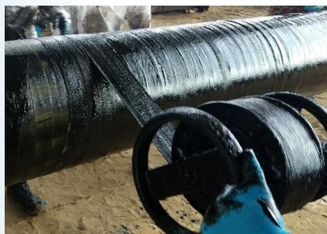
Figure 4: Composite wrapping on progress using specific handles
