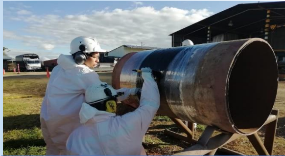
Figure 1: Pipe to be reinforced
