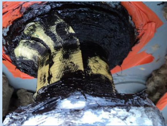
Figure 1: Kevlar® strips application (flare scrubber - part No. 1 of 4.5")
