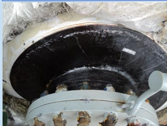
Figure 2: Composite wrapping finished (flare scrubber - part No. 2 of 24")
