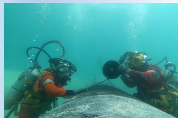
Figure 3: Composite wrapping on progress (step 5)
